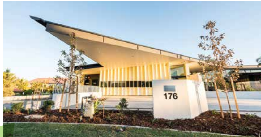
The Asher House development has achieved UDIA certification for sustainable design
